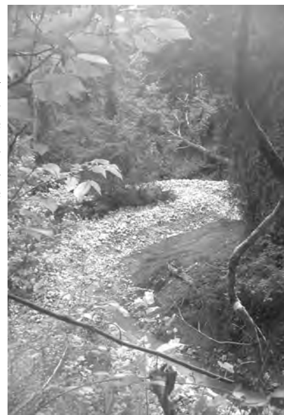
Figure 2: View looking down on the longitudinal peaked stone toe dike in the bottom of Harlin Bayou south of the dormitory.
