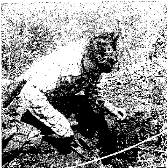
A young Roger excavating at 16OR8, 14 April 1956.
