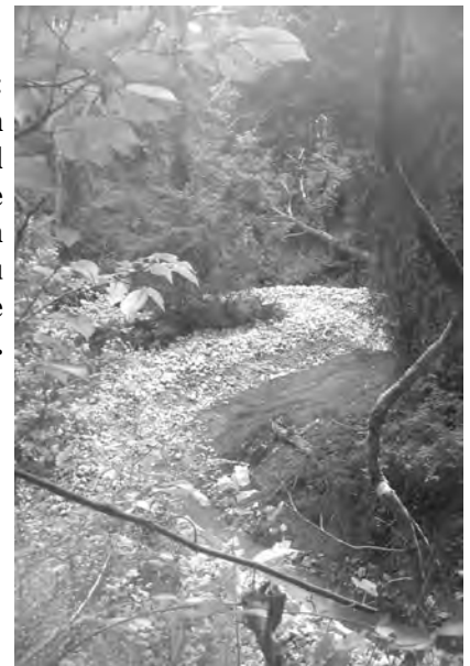
Figure 2: View looking down on the longitudinal peaked stone toe dike in the bottom of Harlin Bayou south of the dormitory.
