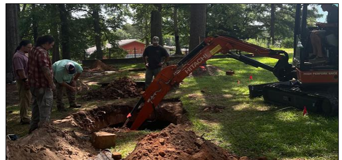
Figure 3. Excavator pulling dirt out of the cistern.
